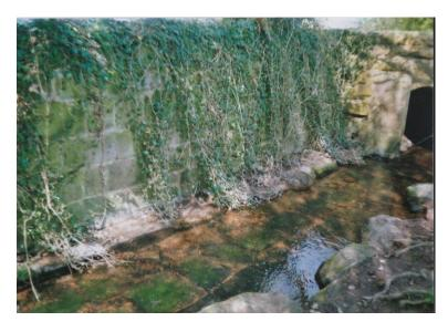
5. 6. and 7. The following three photographs show the stones with slots in them so that boards can be slid into position to dam the water.
